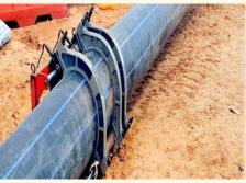
HDPE pipe is butt fused by applying heat to prepared pipe ends and then pushing the pipe ends together with a pre-determined force to make a permanent butt fusion joint with the Hydraulic HDPE Pipe Jointing Machine
